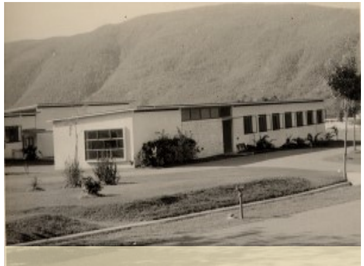
The new ISER building, circa early 1950s. This building currently houses SALISES. Photo Credit: Anne Leaver.
